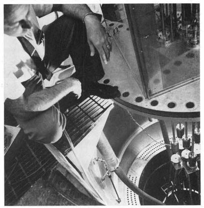
INSIDE OF REACTOR pressure vessel gets a final look by R. M. Jefferson (5331-1). Water now stands 21 ft. deep between the fuel elements and top of the stainless steel vessel, providing an efficient radiation shield. Glass-enclosed mechanism at upper right is for control rods.
